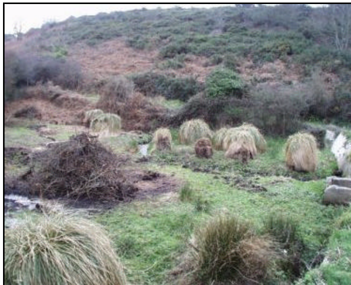
Old Mill leat during clearance work, April 2000
