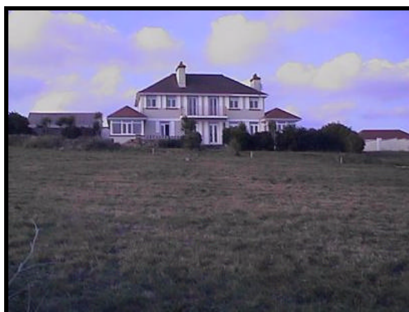
Figure 88. Les Quatre Vents, two days before demolition
