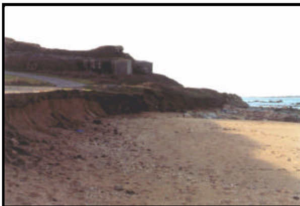
Figure 24. Erosion at Platte Saline, west end.
