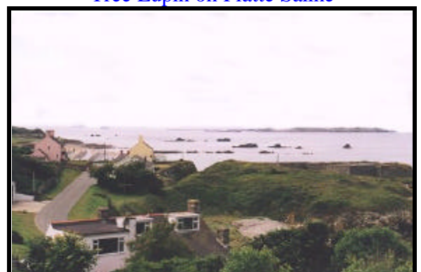
Fort Doyle (on right) and the cutting (centre)
