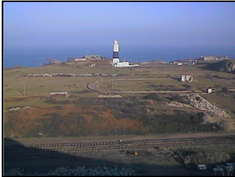
Figure 61. North-east coast with Alderney Lighthouse, Mannez Quarry and Forts Les Hommeaux Florains (L. Centre) and Quesnard (R.), looking north from Mannez Hill
